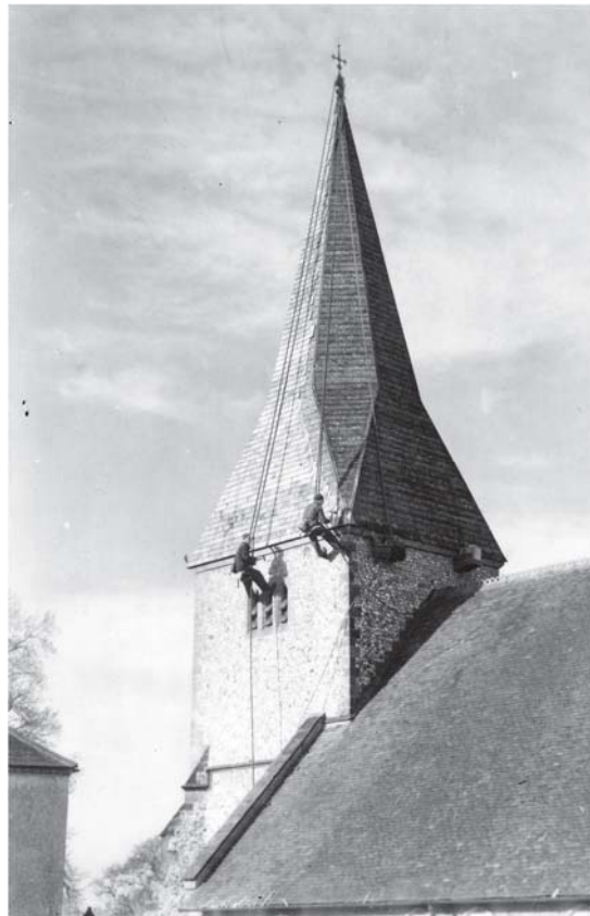
Replacing the Shingles, 1954 by George Garland (© WSRO 3128A)
