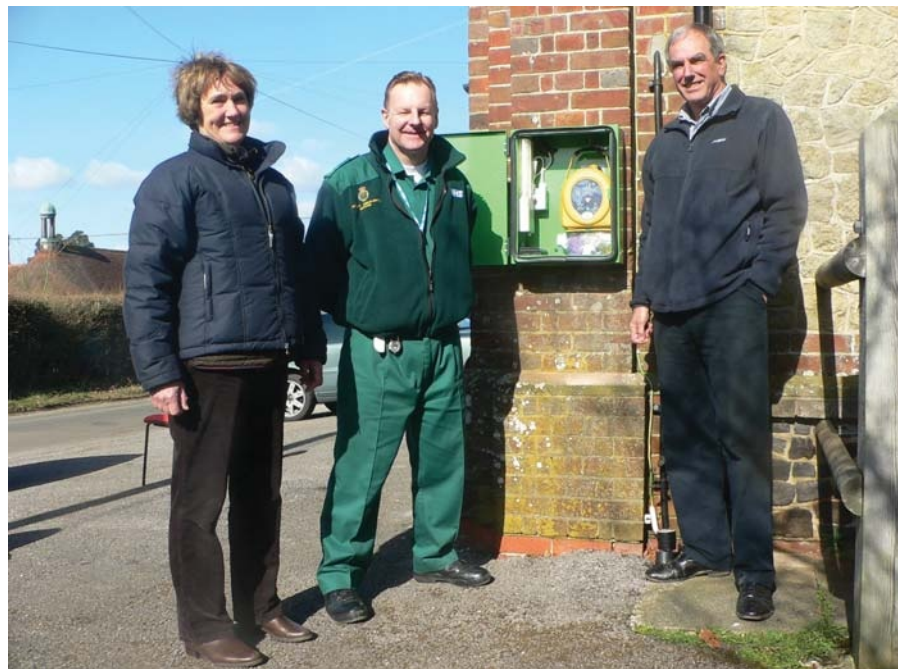
Installing a defibrillator at the Empire Hall - Alison Davidson with a trainer from South East Coast Ambulance Services and Roger Coakes
