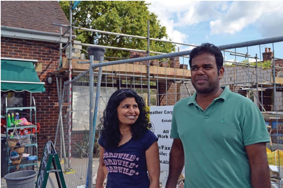
Building work in progress, 2015
