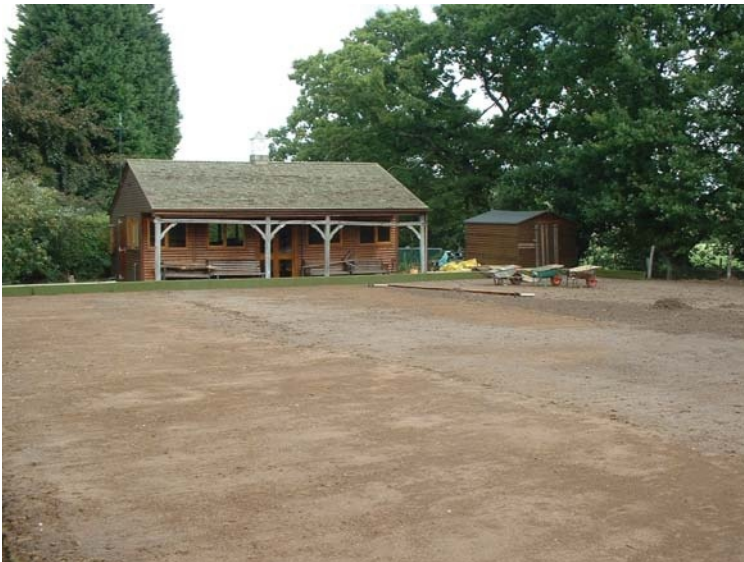
Below: Replacing the Green, 2007
